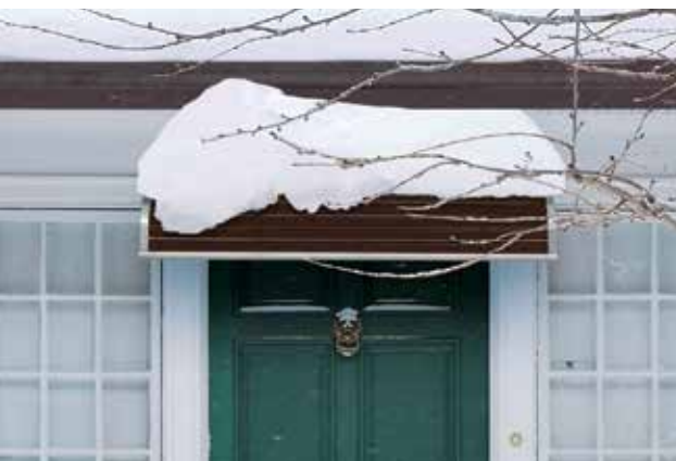
SNOW: Door canopies help protect your entryway on harsh winter days helping to reduce ice and snow from steps and landings.
